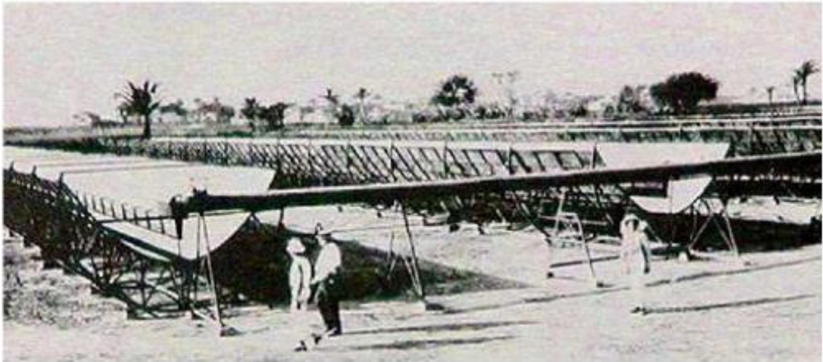
Frank Shuman parabolic solar collectors, Maadi, Egypt, 1912
